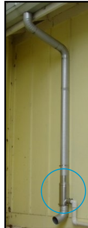
Fig. 9: Downspout filter
