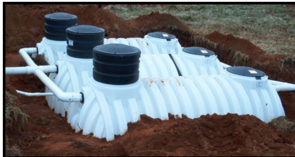
Fig. 8: Below ground tank
