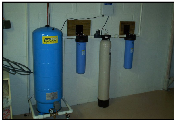
Fig. 15: Residential UV light potable water treatment Photo courtesy of Rainwater Management Solutions.
