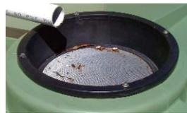
It is important that roofs, gutters, screens and first flush devices be inspected and cleared of leaves and other debris every three to four months.
