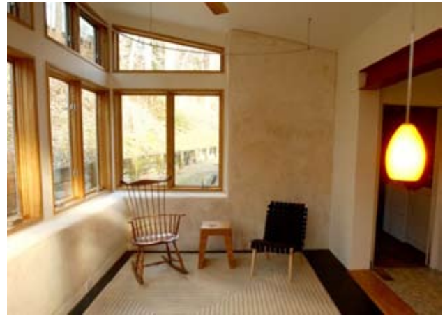
Straw Bale Walls finished with Lime Plaster
