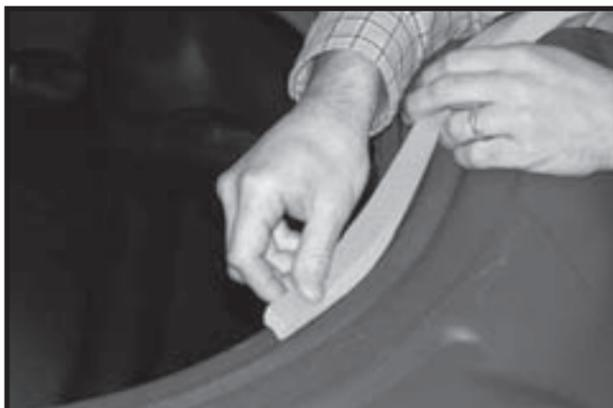
**FIG.2 Apply Gasket**
