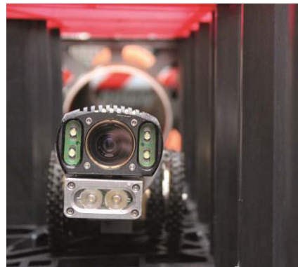
Inspection with camera
