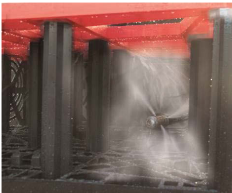
Jet washing the system
