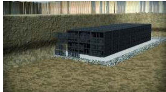
Once all the blocks are positioned, the system is fully wrapped in **geotextile**. This prevents the ingress of dirt particles into the system.
