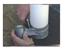
Seal base of pipe with adhesive tape and silicon.
