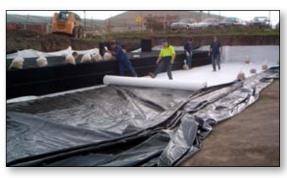
Use pins, rocks or sandbags to prevent geotextile from sliding or blowing down into the excavation.
