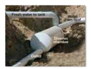
The Rain Harvesting In-Ground 12" First Flush water diverters improve rainwater quality and safety, help extend the life of pumps (used to distribute rainand internal appliances that draw upon rainwater (such as laundry, toilets, hot water systems and dishwashers) and reduce tank maintenance.
