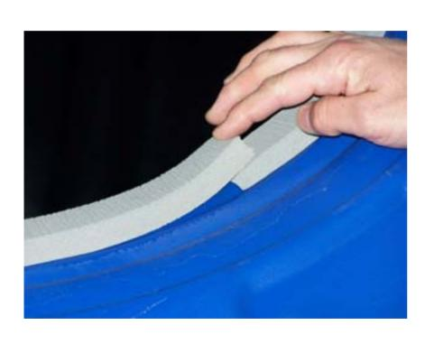
A properly trimmed gasket is then compressed end to end
