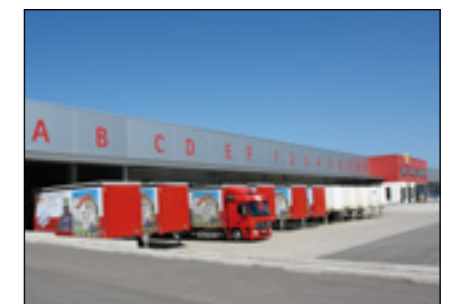
Teningen logistics centre
